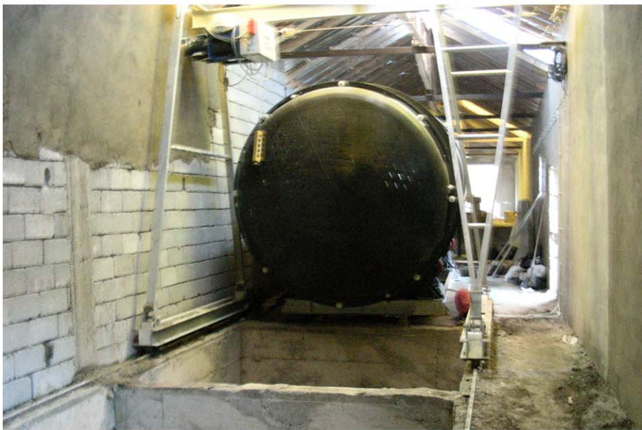
ÇATAK (VAN) SOLID WASTE COMPOSTING PLANT Views during construction and erection of equipment.
