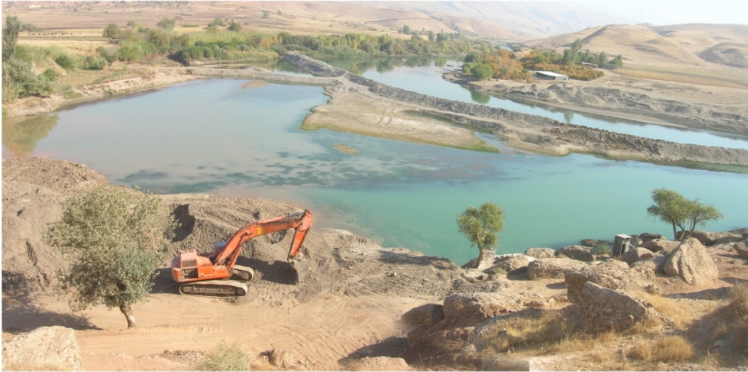
Diversion of the river.
