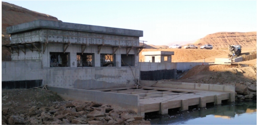
Construction of Intake and Pump Building.
