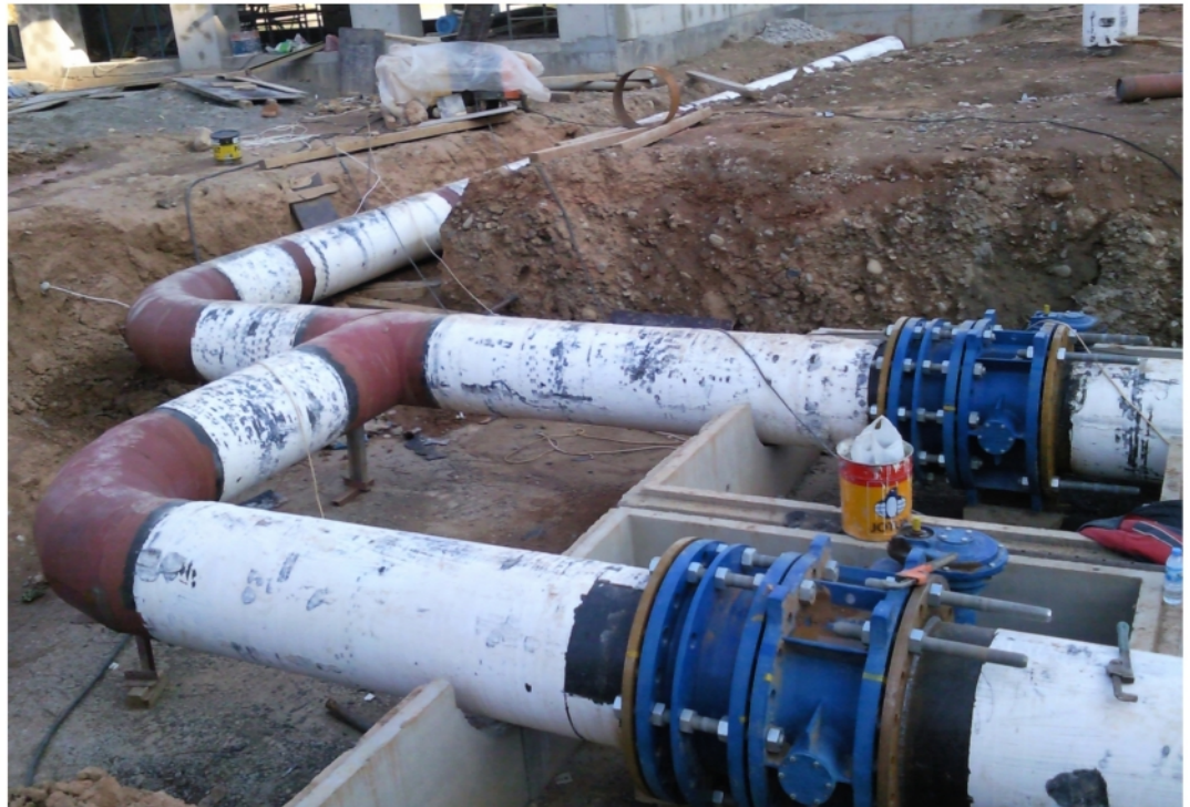
Installation of pipes, valves and flowmeters.
