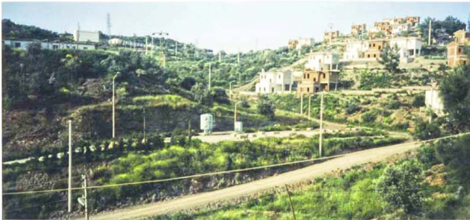
SEMIRAMIS HOLIDAY VILLAGE (BODRUM) WASTEWATER TREATMENT PLANT (1.000 m 3 /day)
