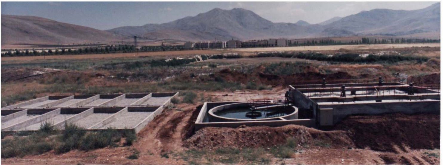
ELBISTAN SUGAR FACTORY DOMESTIC WASTEWATER TREATMENT PLANT (500 m 3 /day)
