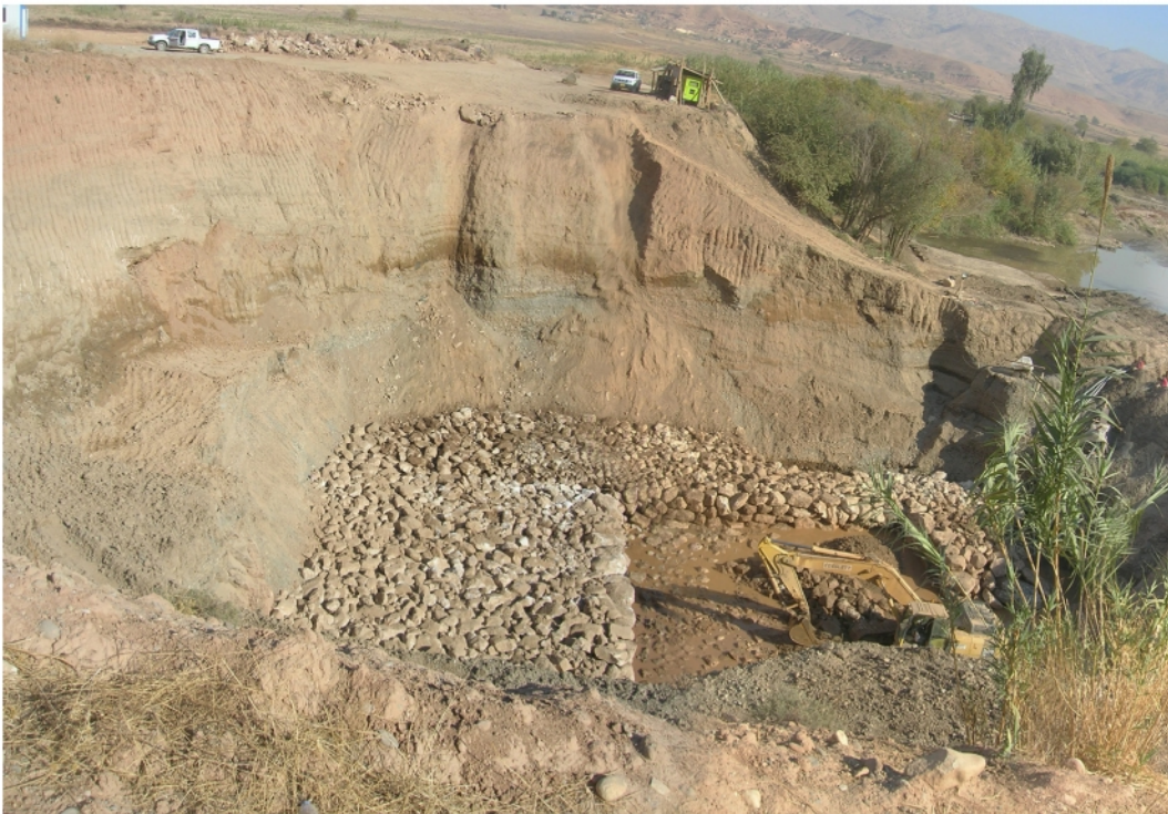
Excavation and rockfill at the foundation.
