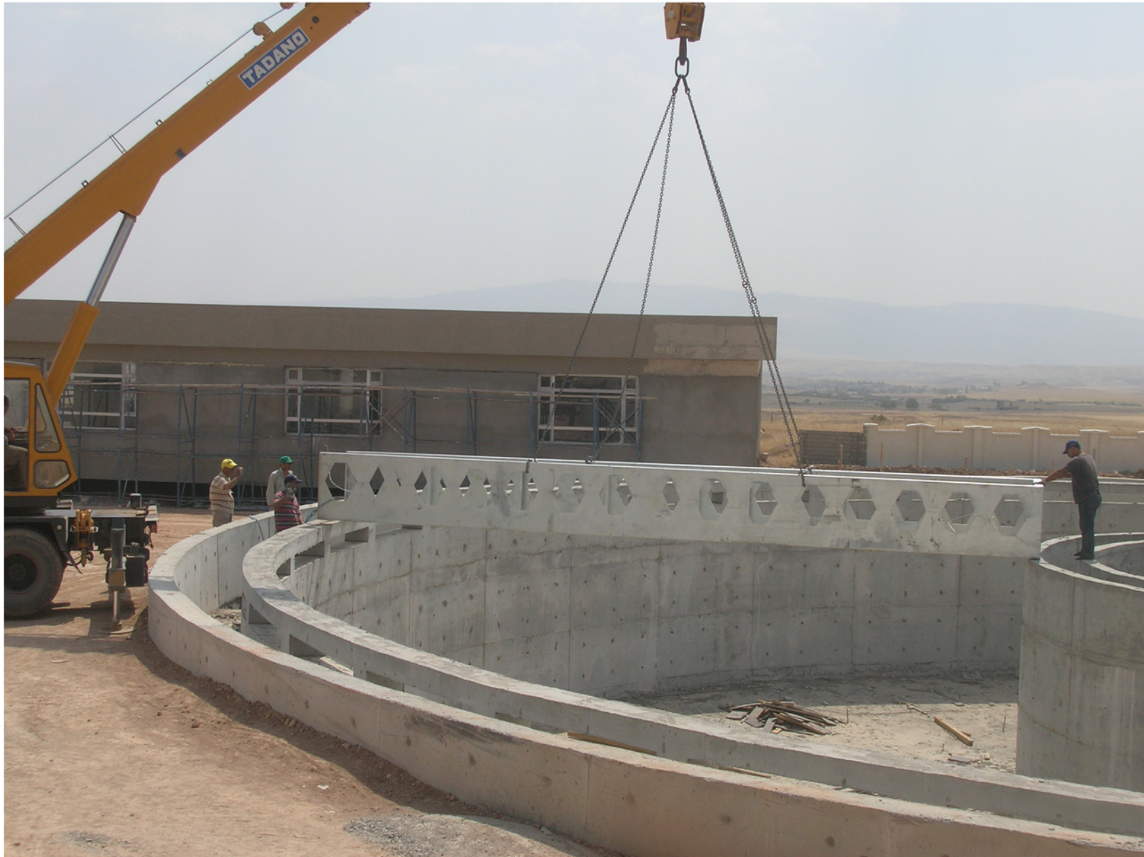
Scraper bridge during erection.
