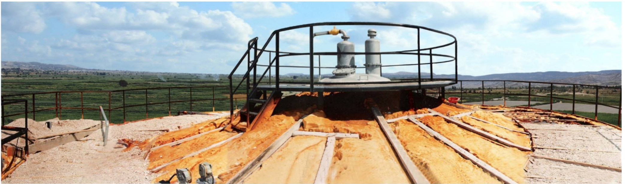
View of the Top of Anaerobic Reactor During Construction Showing the Insulation Details, Gas Dome, Flame Arrester, and Vacuum Break.
