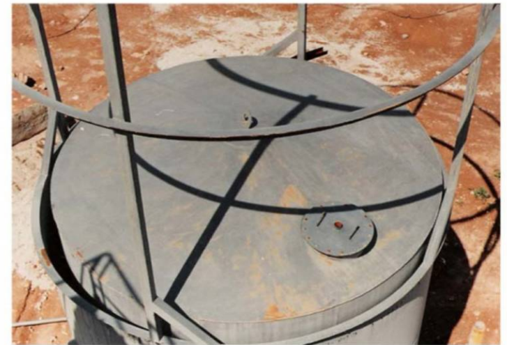
View of the Gas Storage Tank During Construction
