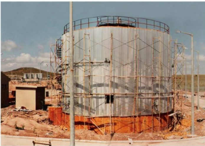
View of the Anaerobic Reactor During Construction
